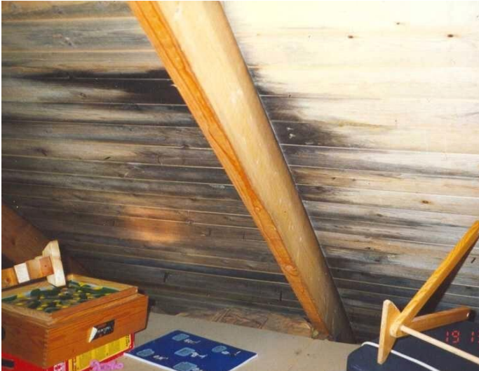
Figure 1. Mould growth in a cold attic.
